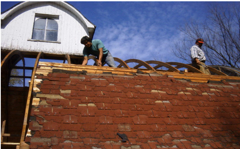
corn crib undergoing transformation, 2003
